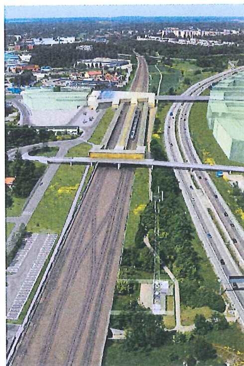
Barkarby station, etapp 2
