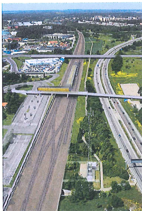
Barkarby station, etapp 1
