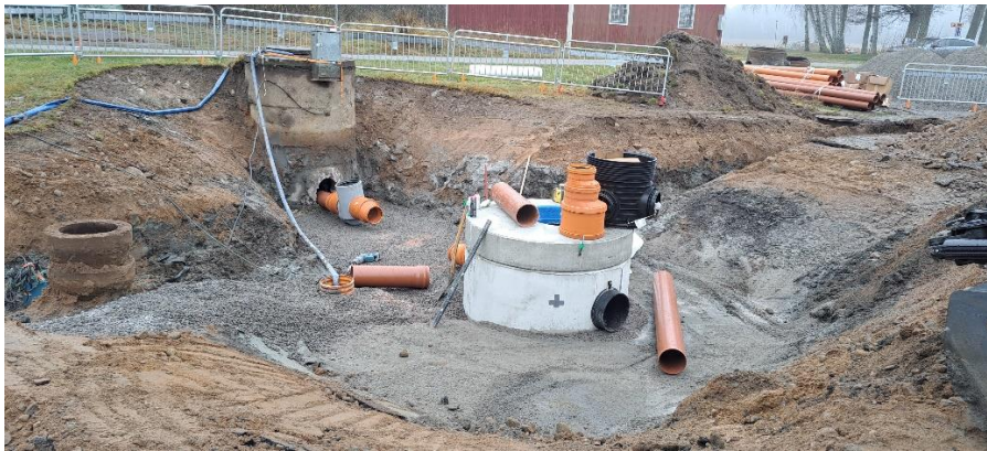
Figur 7: Oljeavskiljare under installation
